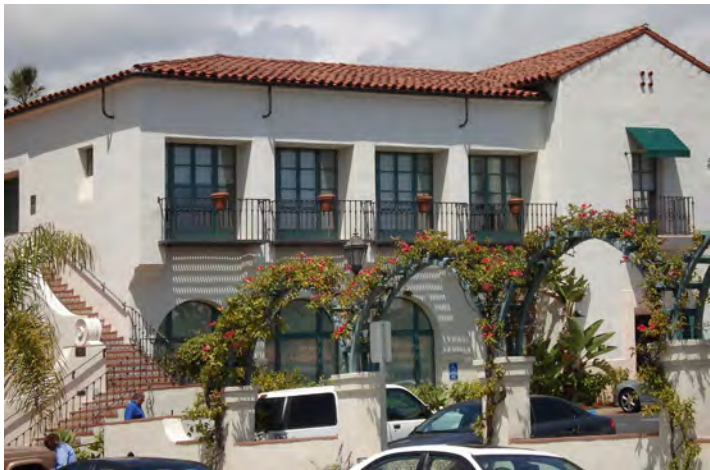
Figure 6-33 - Windows (6.10.5) Windows are recessed from the exterior wall surface.
