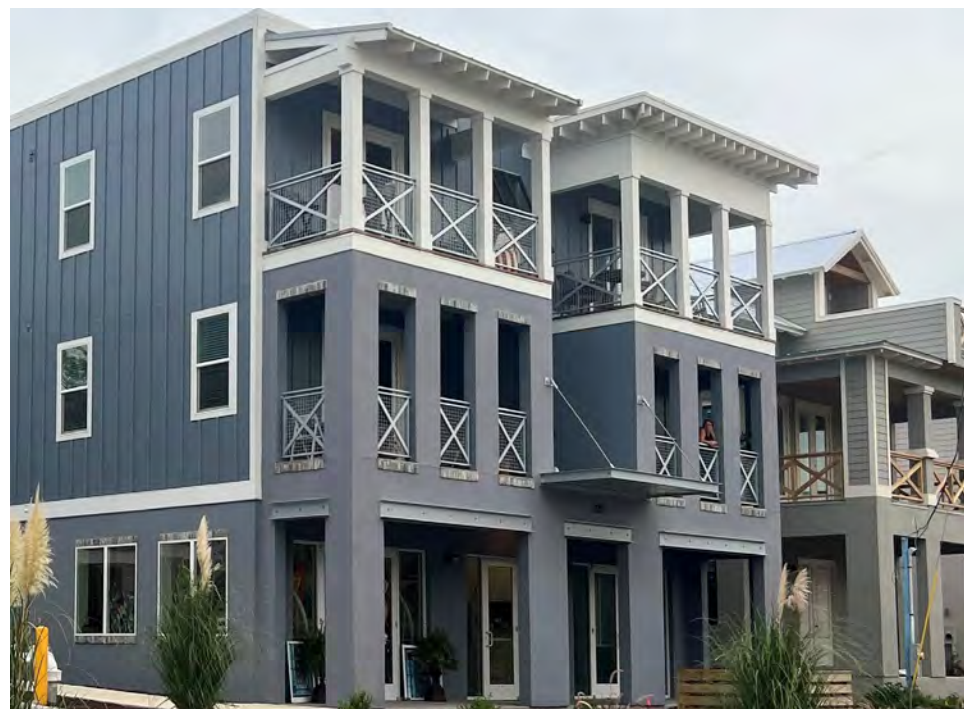
Figure 6-17 - Walk-Up Building Illustrative Photo
