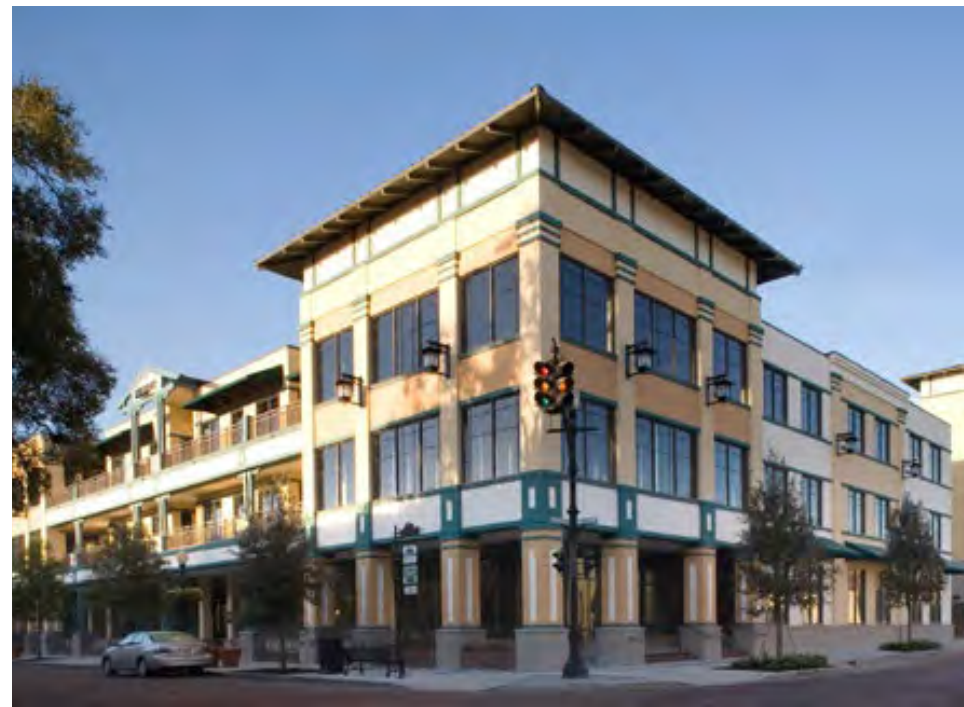
Figure 6-23 - Liner Building with Garage Illustrative Photo Street view of a liner building. The facade does not reveal the parking use behind.
