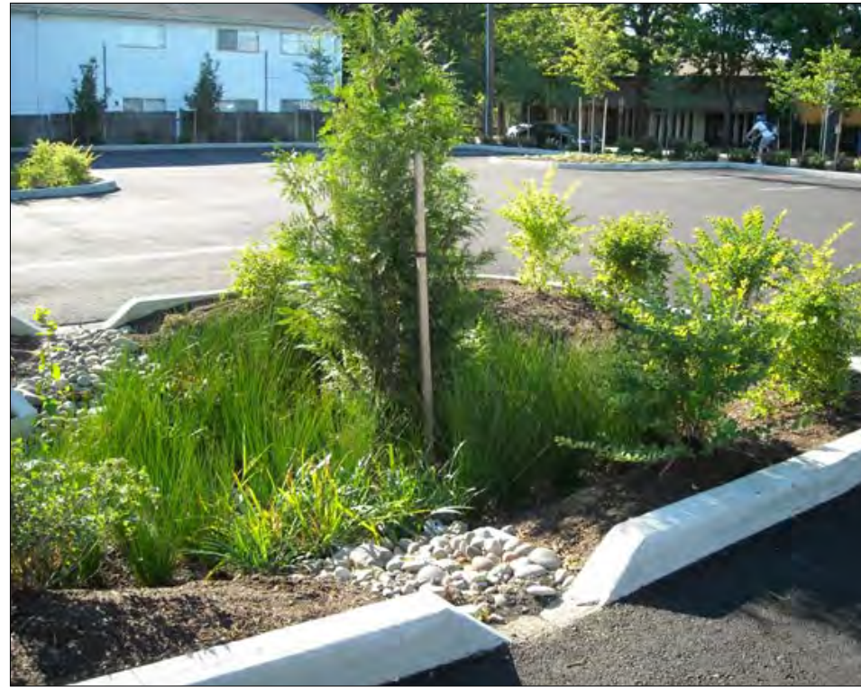
Figure 3-35 - Curb cuts allow water to flow from a parking lot into a planted bioswale
