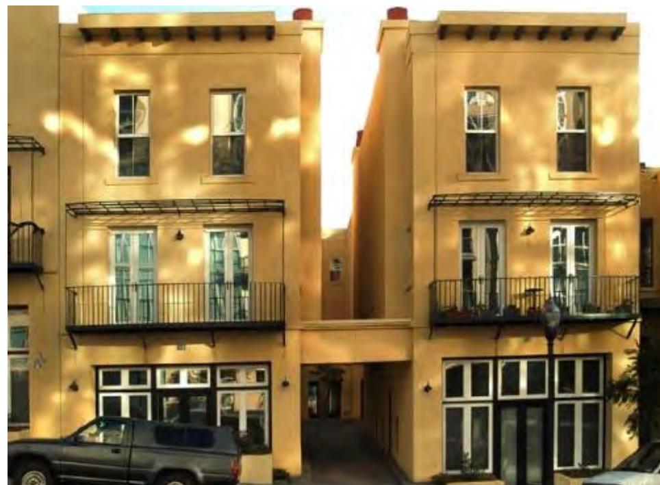
Figure 6-15 - Flex/Loft Building Illustrative Photo
