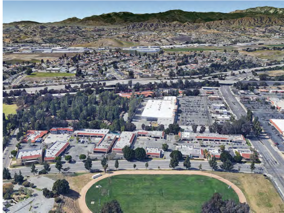
Figure 1-8 - View looking North West (Blocks West of Diamond Bar Boulevard)
