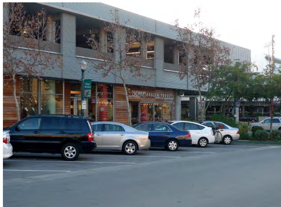
Figure 6-29 - Exposed Garage Building Illustrative Photo
