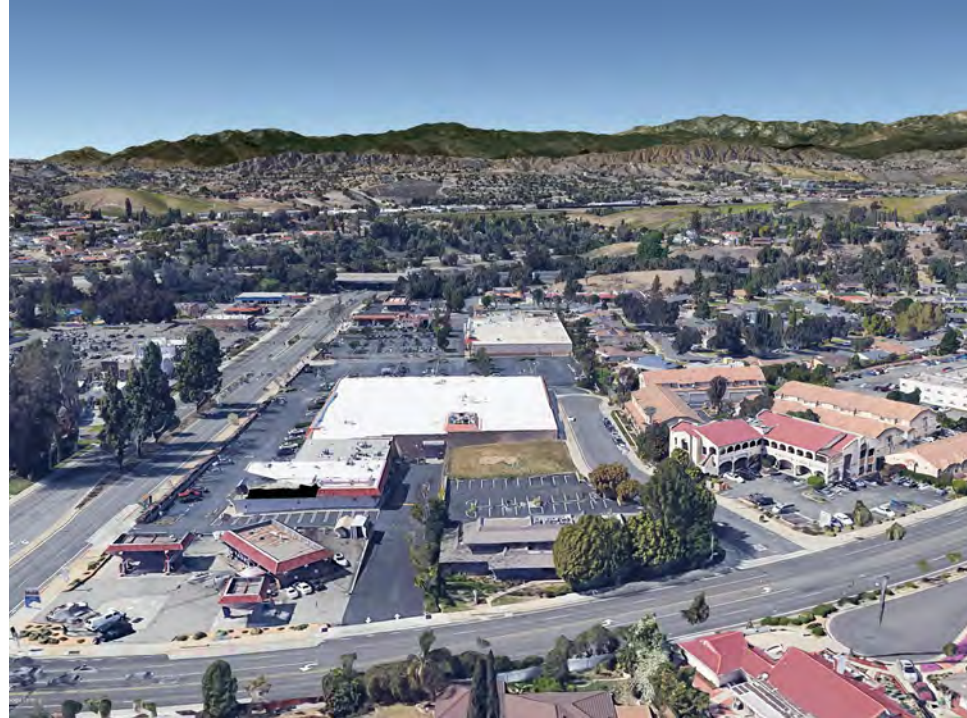
Figure 1-10 - View looking North West (Blocks East of Diamond Bar Boulevard)
