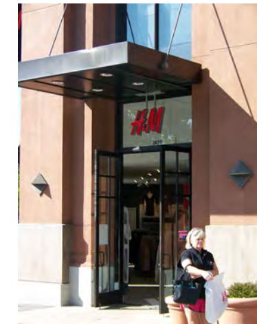
Figure 6-32 - Entrances (6.10.4) A canopy, lighting, and a slight recess accentuate the primary entrance.
