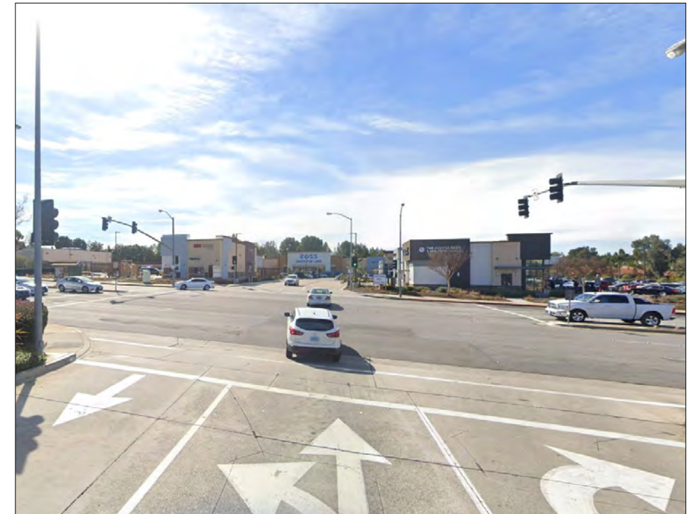
Figure 1-21 - Existing wide intersection
