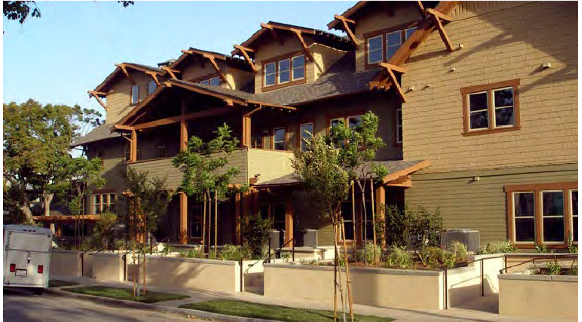
Figure 6-91 - Craftsman Style Building - Fair Oaks Court, Pasadena, CA
