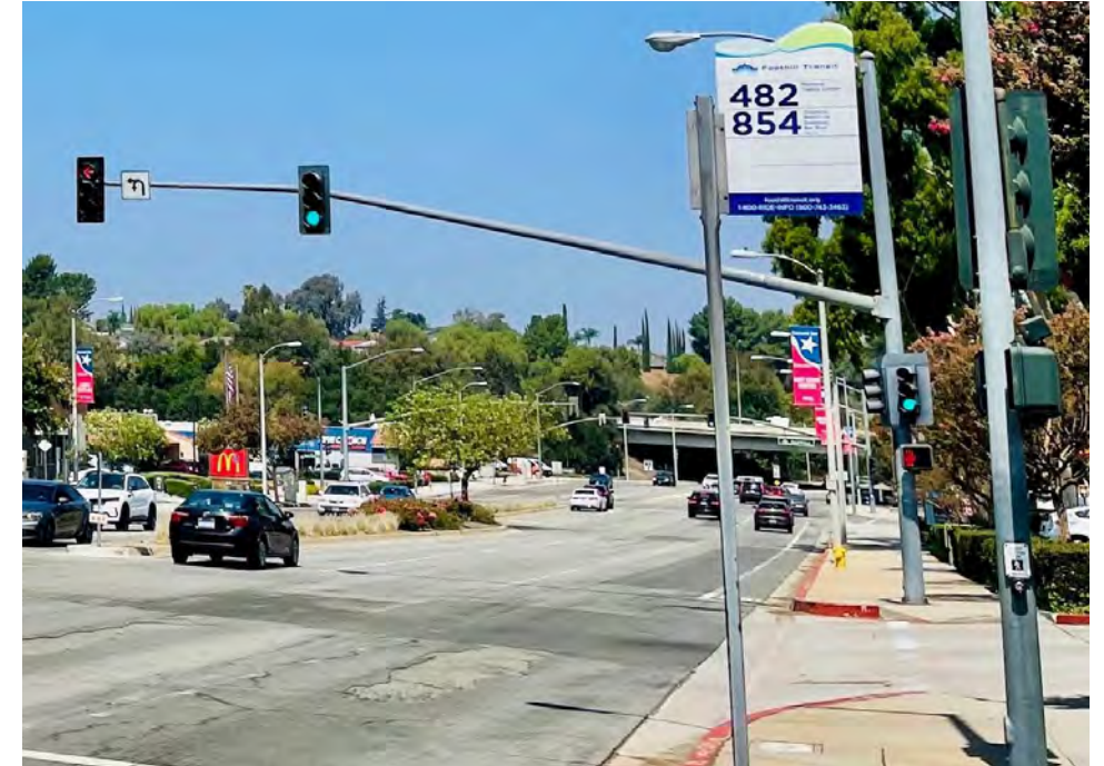
Figure 3-9 - Narrow sidewalks interrupted by utility poles
