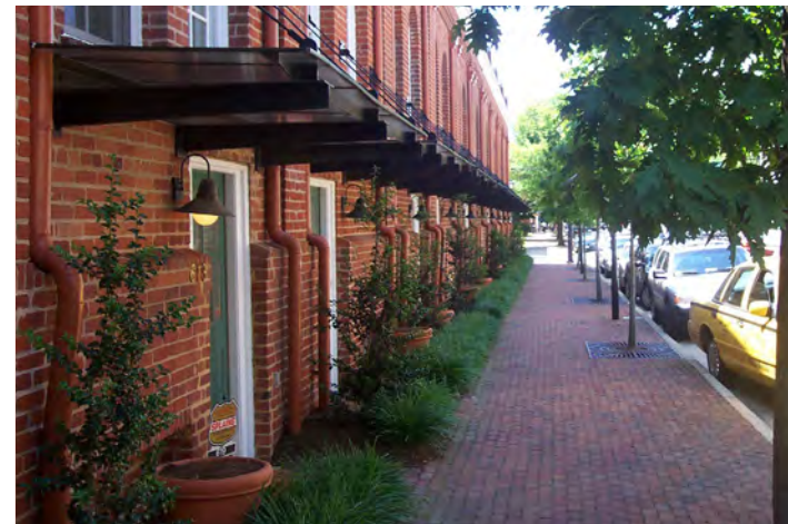
Figure 6-36 - Projecting Canopies (6.6.8) Canopies create a rhythm along the streetfront and accentuate the building entrances.
