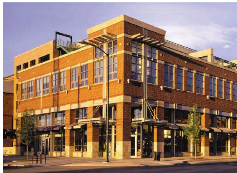
Figure 6-21 - Urban Block Building Illustrative Photo
