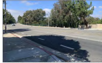
3 Sidewalk connects pedestrians to Sycamore Canyon park and wildlife area
